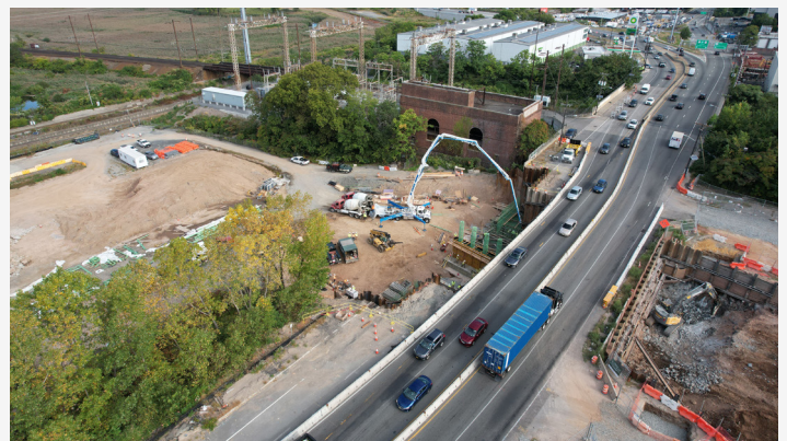
Tonnelle Avenue Bridge & Utility Relocation
