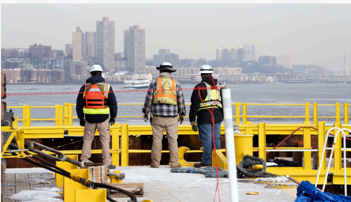
Hudson River Ground Stabilization
