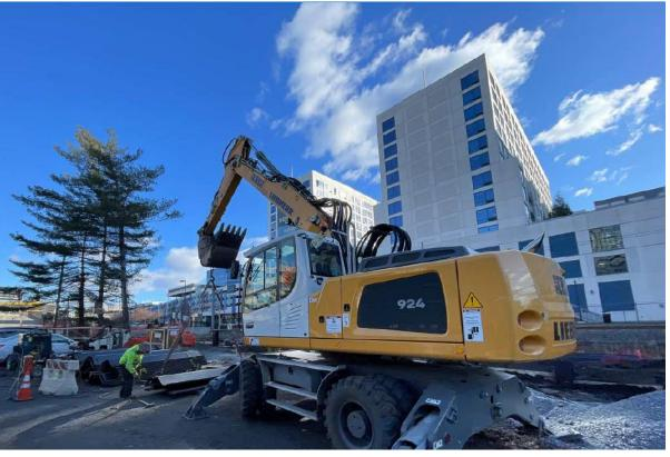
Preparatory work is in progress, including erosion control measures, rock and environmental borings, clearing, and monitoring instrumentation installation. Haul route construction is expected to begin at the end of February.
