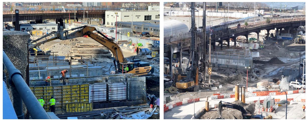
Secant pile installation will be finished before the end of the year. Once complete, excavation to install the tunnel box will begin.
