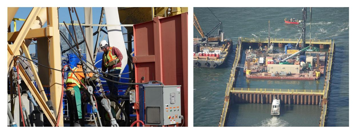
King pile and sheet pile installation for the first 600 feet of the cofferdam was completed ahead of schedule. Deep soil mixing and coring samples are now underway.
