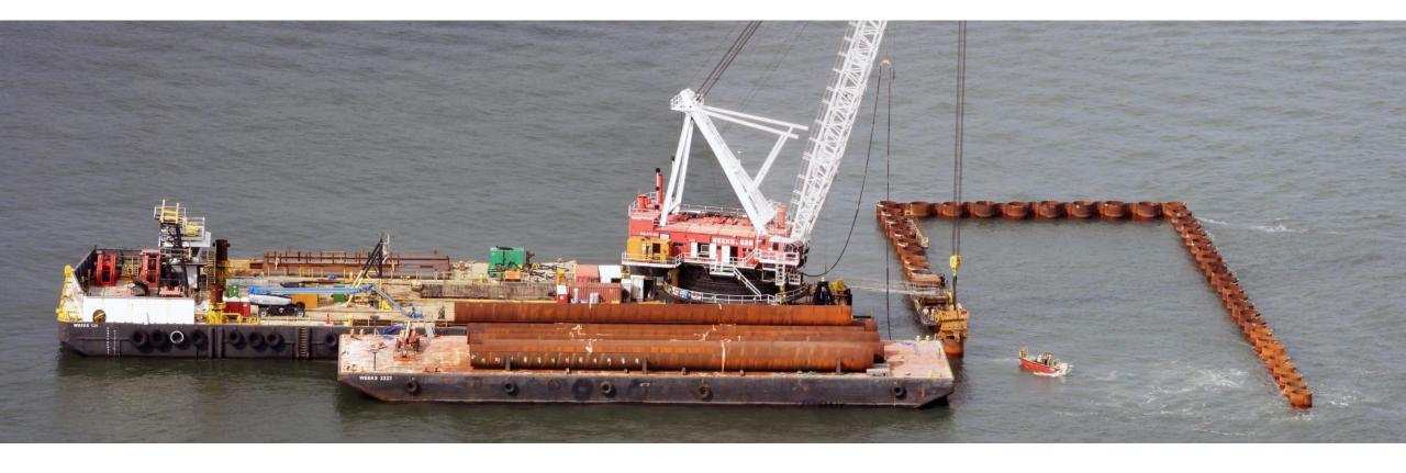
King pile and sheet pile driving for the test section is finished. Acoustic corer scans are roughly 50% complete.
