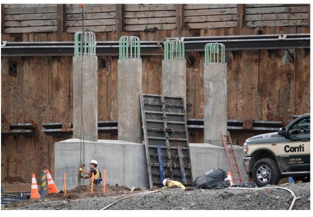
Concrete has been poured for the northwest abutment footing, wingwall footing, and center pier crash wall. Permanent sheeting to support the right-of-way walls is nearly complete.
