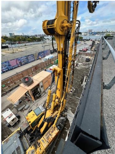
Secant piles are more than 65% complete and work has started on underpinning the High Line.
