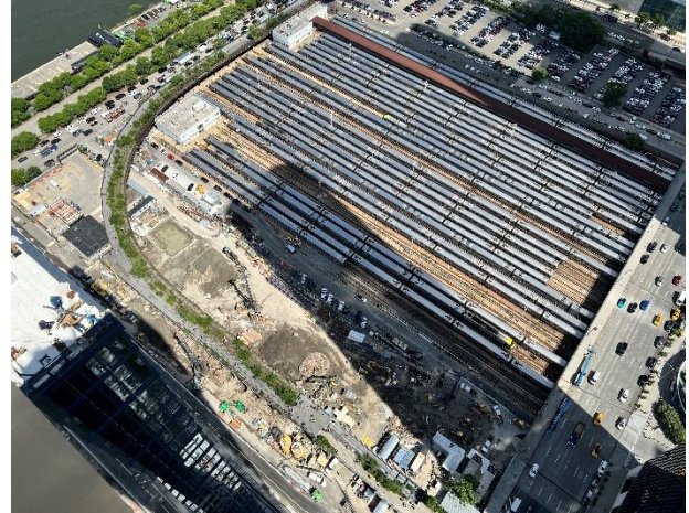
August 2024 construction progress at HYCC-3
