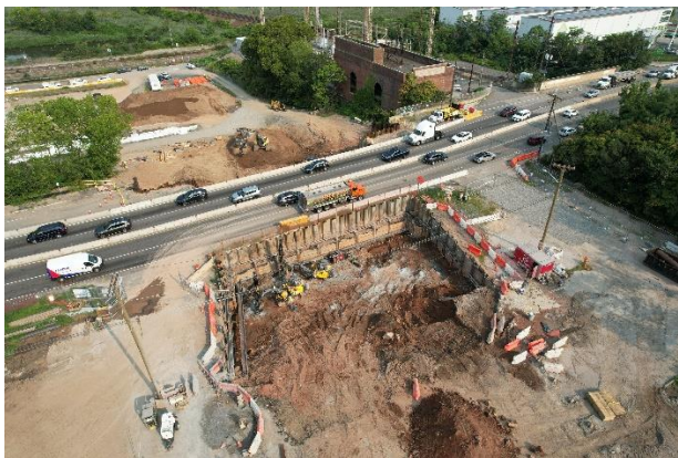
Shoring work on the eastern side of the Tonnelle Avenue Project
