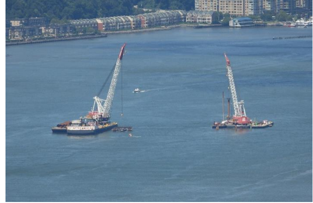
HRGS floating construction barges
