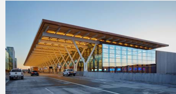
New Kansas City International Airport City of KC – Edgemoor/Clark - $1.5B - 2023
