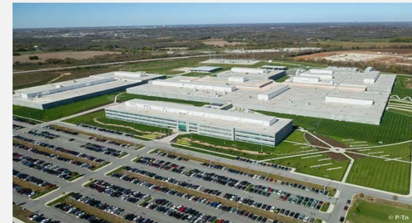
National Nuclear Security Administration Campus Kansas City, MO GSA - JE Dunn/HNTB - $1.0B - 2012
