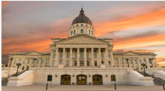
Kansas State Capital Renovation, Topeka, KS State of KS - JE Dunn - $600M - 2011
