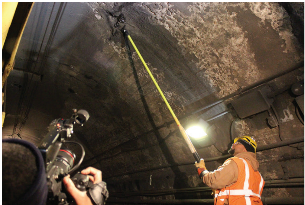
De-icing in the Existing North River Tunnel
