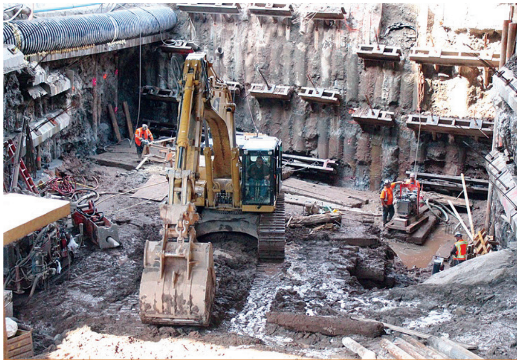
Section 1 of the Hudson Yards Concrete Casing under construction in 2014.
