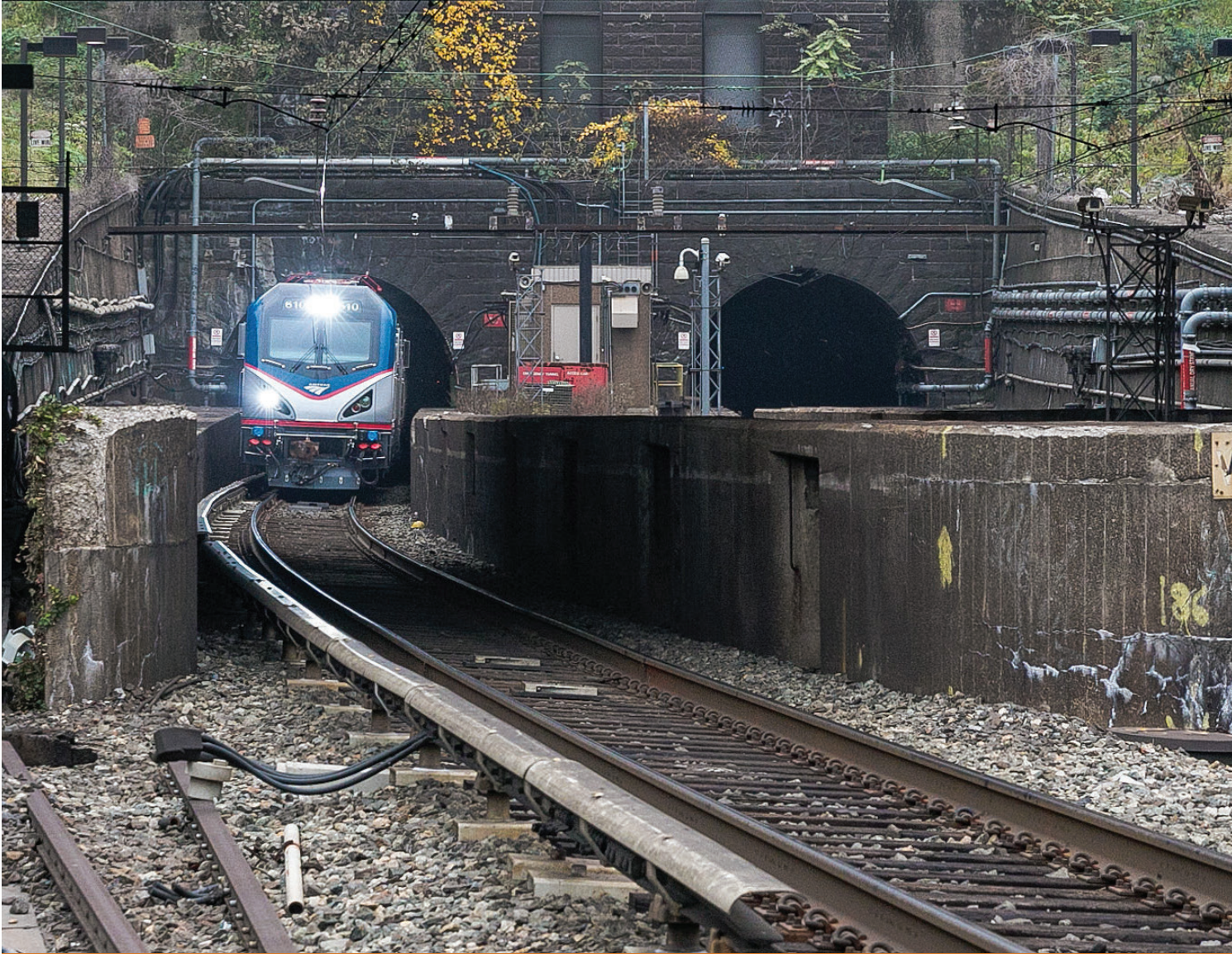
Existing North River Tunnel in New Jersey
