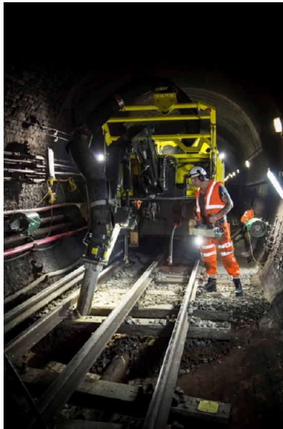
Figure A10.12: Baker Street to Finchley Road ballast removal
