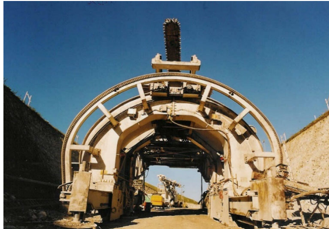
Figure A10.4: Pre vaulting tunnelling machine Ramsgate Port Access tunnel
