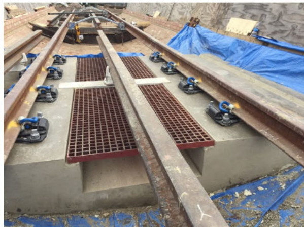
Figure 10-4: LUL Baker Street to Finchley Road Mock-Up Trials
