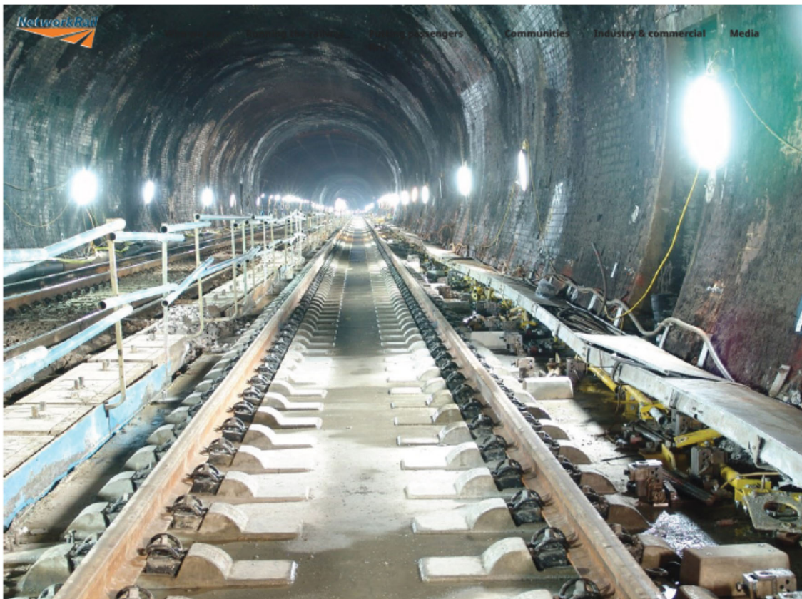
Southampton Tunnel, UK, during 12-day outage to install 1600 ft long slab-track.
