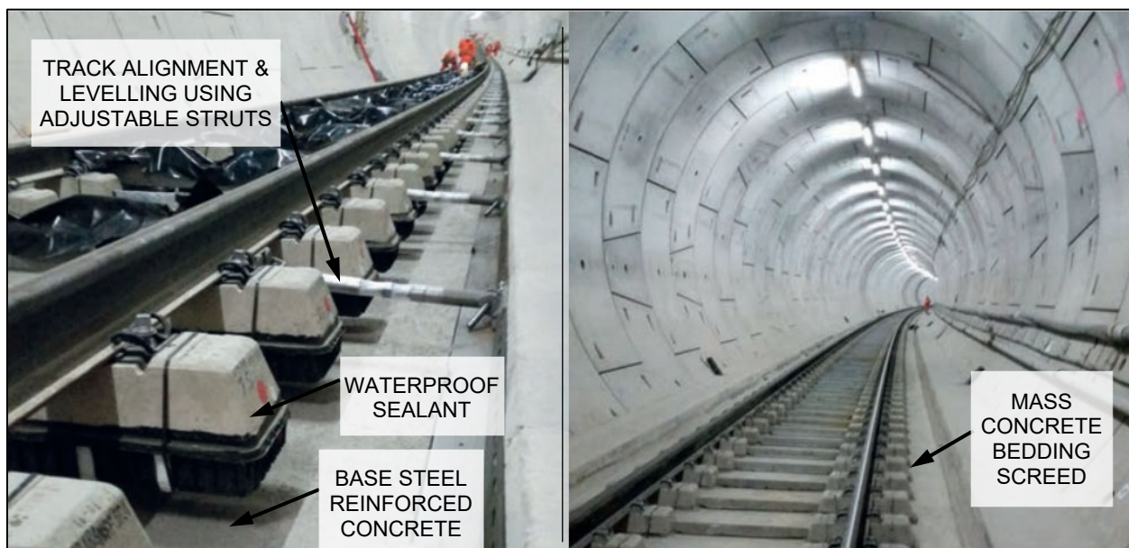
Figure A6.2 Key elements of the booted track tie system
