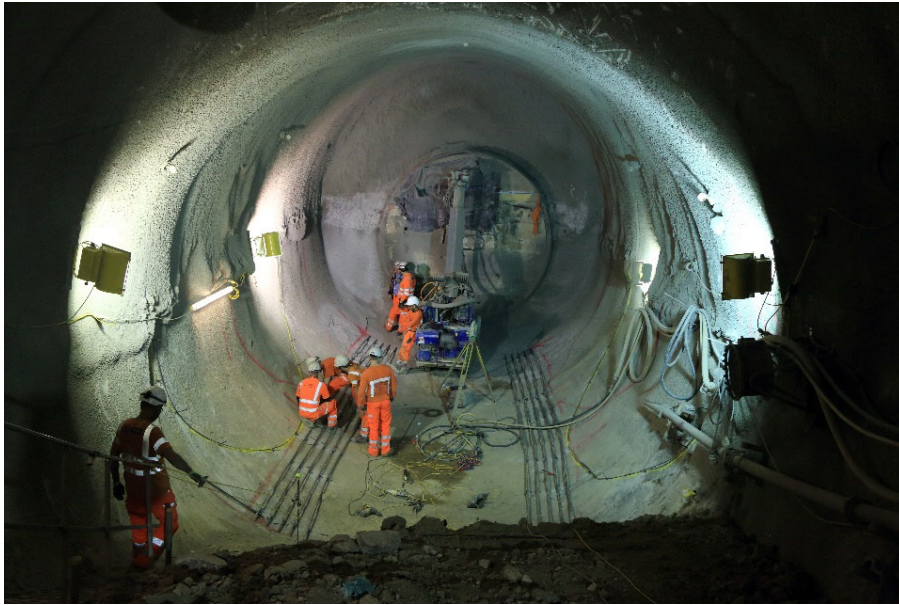
Figure A10.7: Bond Street Station Upgrade below ground works
