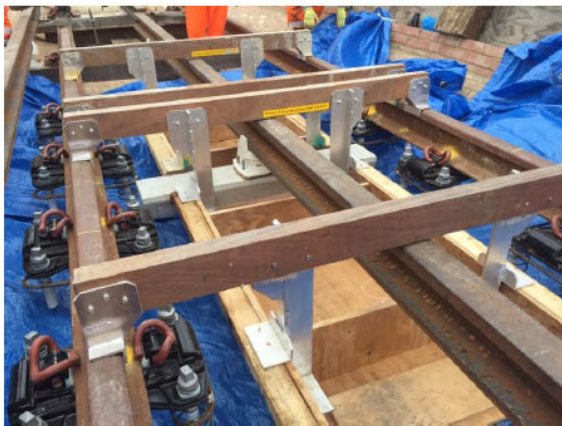
Figure 10-3: Mock-up built to trial method and develop concrete mix and concrete finish for Slipform paved Haunches for HS1 London Tunnels Alliance
